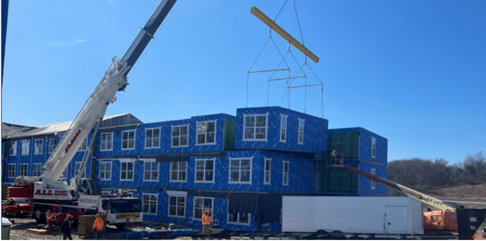
Setting of Last Module on Building 1 (January 2024)
