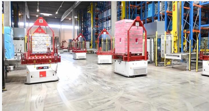
Automated Pallet Delivery Systems
